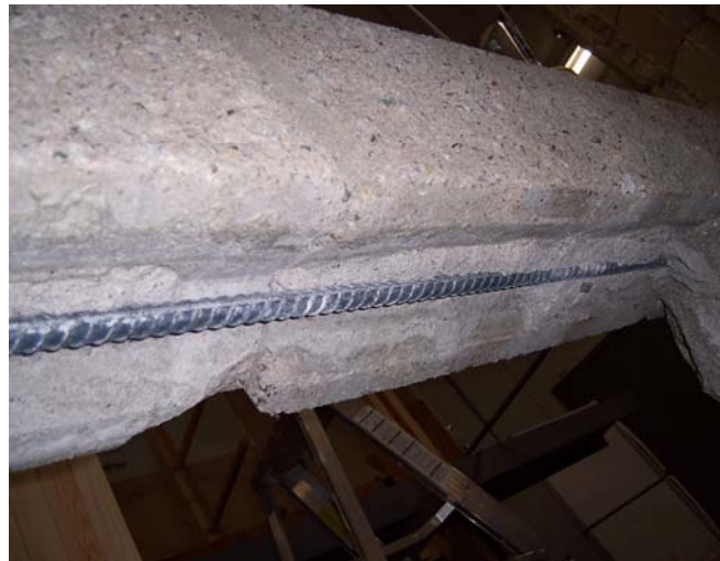
Figure 3: Horizontal Bond Beam Steel after demolition
