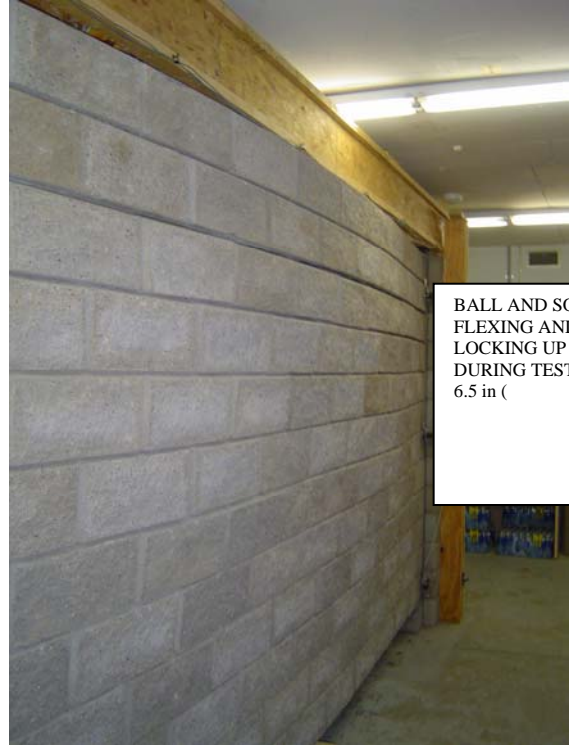
Photo A4: Panel During Stressing
